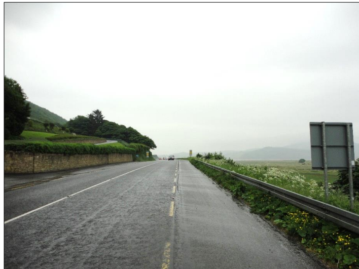
Extended Pinch Point along the R238, looking towards Fahan.
