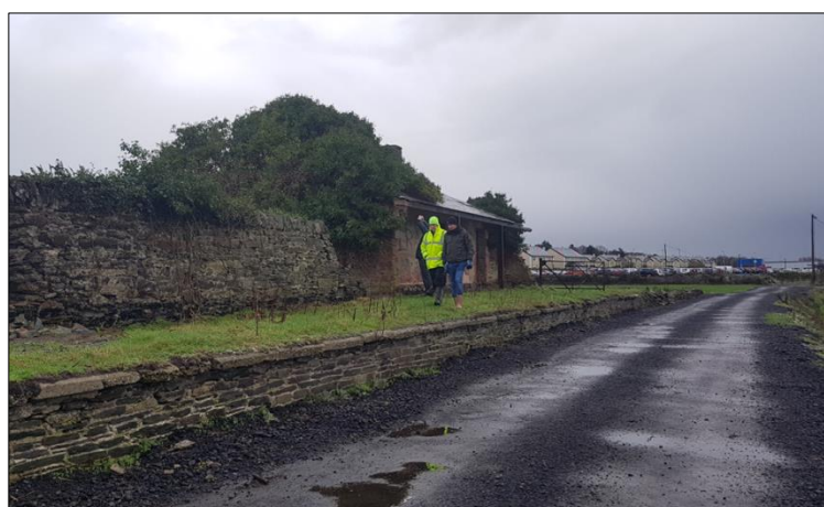
Old Station House, at railway line (currently farm lane, looking back toward Slab Road.
